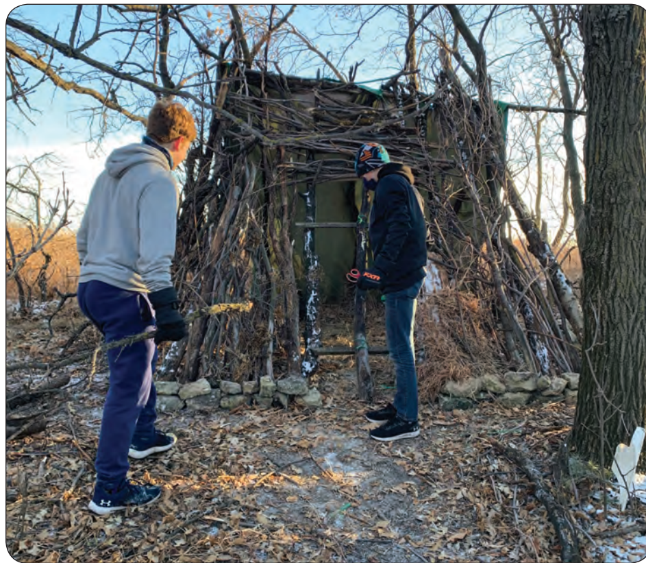
STANDARD PHOTOS SUBMITTED Starbuck School Phys Ed teacher Tim Morison's students work together to build a shelter.
