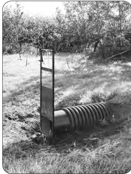
In the Morris Norquay Sub-District, Alan Richardson installed a gated culvert with help from the RBWD to regulate wetland water levels.
