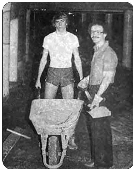
Don McKibbon and Marsh Kennedy "dig in" to get the underground track completed.
