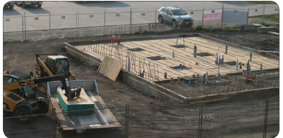
The Tim Hortons walls started going up this week.
