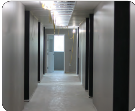
The hallway on floor three.
