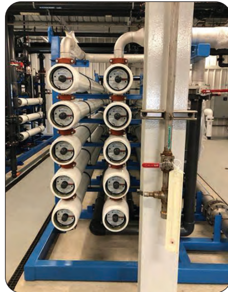
The Morris water treatment plant also saw improvements, including a new membrane skid addition.
