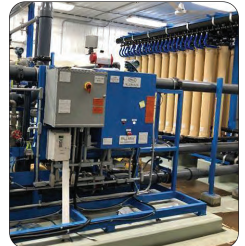
The Morris water treatment plant also saw improvements, including a new membrane skid addition.
