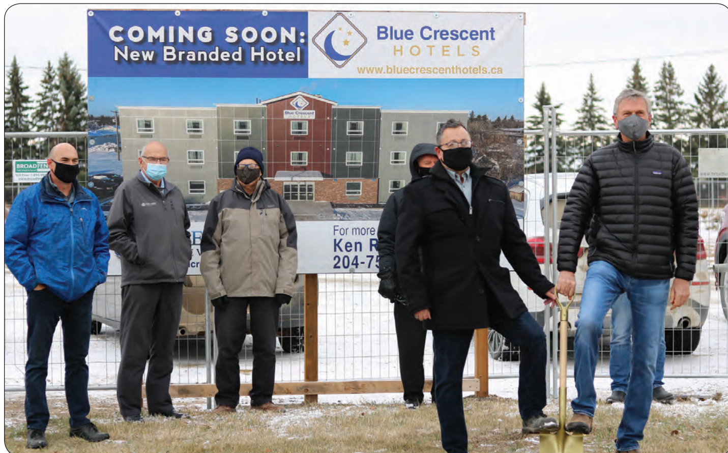
Construction on the Carman hotel has officially started.
