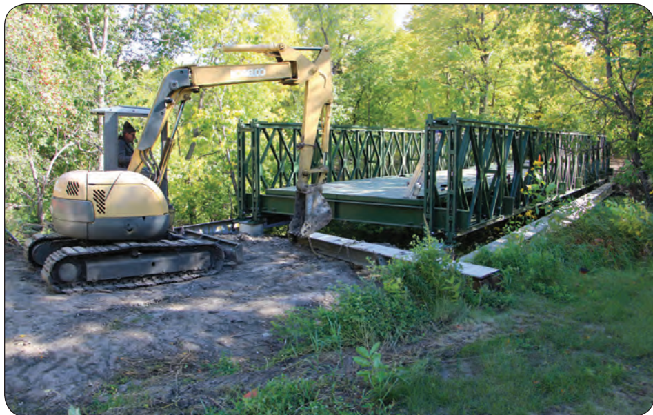
Reimer plans to finish the bridge completely before winter.
